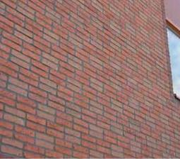
You can be very creative with brickwork bonds. Here the block bond has 4 courses, but it alternates with a horizontal-vertical stack bond.
